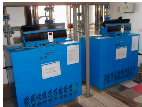
a) hot water boilers of the hot water circuit
